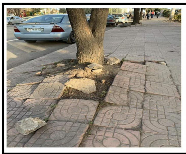
Figure 8: Roadside trees conflicting with sidewalk and electric power line
